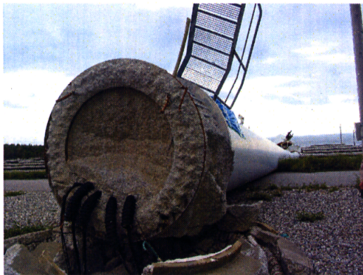
Fig. 3. Destroyed wind turbine by typhoon in Miyako-jima isaland, Okinawa
